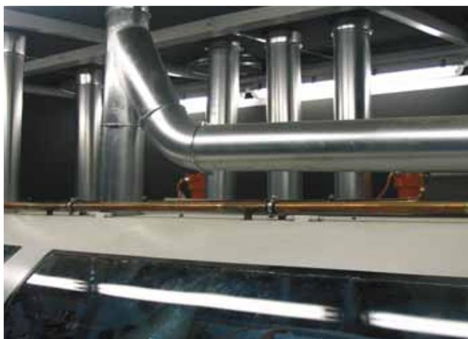
Firefly's PlanerGuard system *detects* sparks or incipient fire *at a very early stage*. The PlanerGuard system can be designed in a cost-efficient way due to the compact design of the moulder. *Water mist* will extinguish quickly and efficiently, even in these closed areas. Water mist also ensures that your moulder isn't damaged by water.
